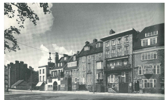
Cheyne Walk - built project, photo 1897
